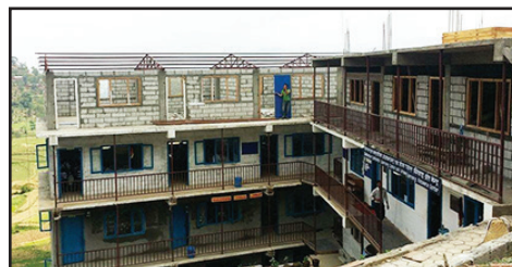
School under construction in Pharping, Nepal
