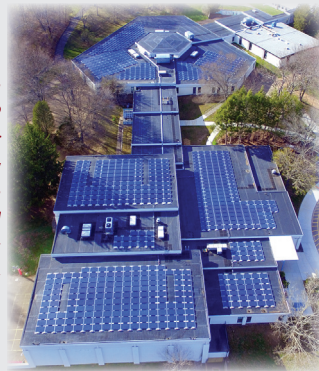
Beecher's blue roof? 970 solar panels now produce one-third of school's electricity - pg 11
