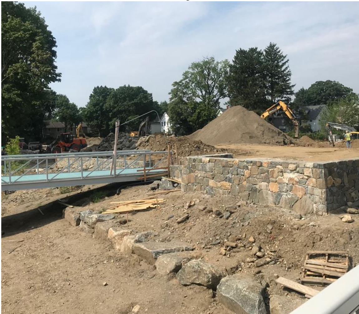
Site activities looking South – 7/31/19
