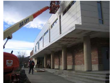
Sandstone used for the veneer, was recycled from the existing building
