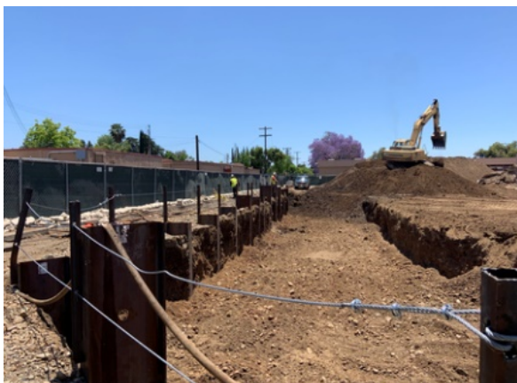
Setting steel beams, guide wire and lagging.
