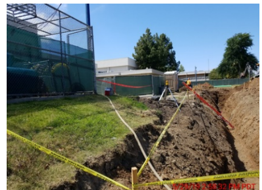
Excavation of underground routes
