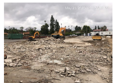
Building 300 demolition completed. Rock bed encountered in the excavation. Construction debris being set aside and hauled daily.
