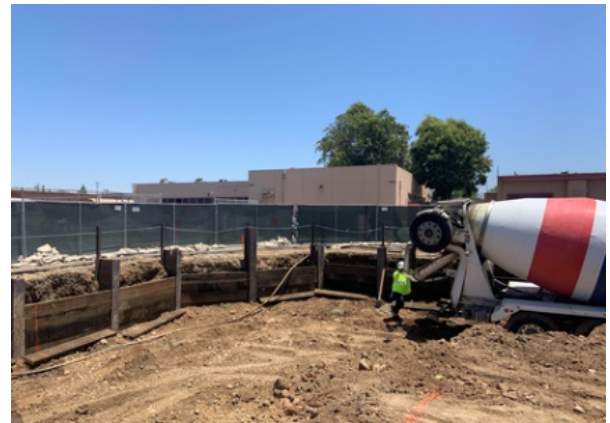
Over excavation of the new science building location.
