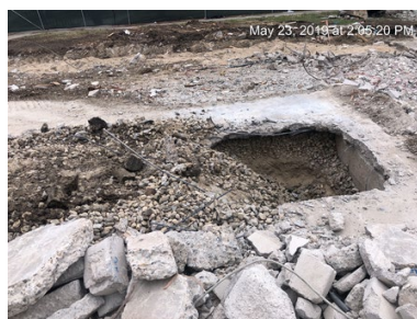
Building 300 demolition completed. Rock bed encountered in the excavation. Construction debris being set aside and hauled daily.
