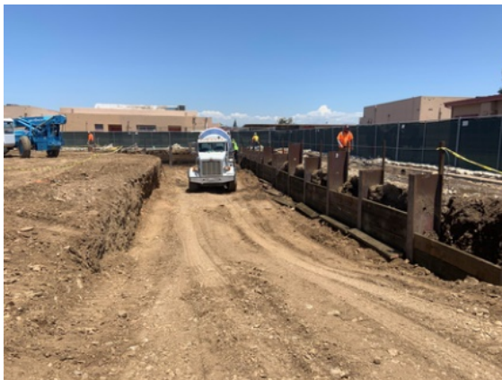
Over excavation of the new science building location.
