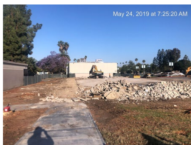
Building 300 demolition completed. Rock bed encountered in the excavation. Construction debris being set aside and hauled daily.
