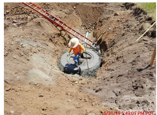
Excavating and setting manhole in trench.
