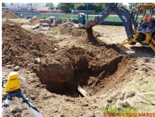
Excavation carefully while uncovering pipes.
