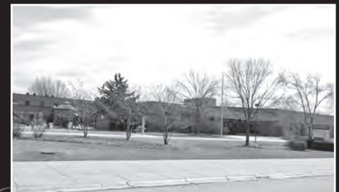
Waterbury Elementary School
