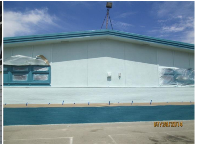
Fisher Exterior Repair/ Paint project
