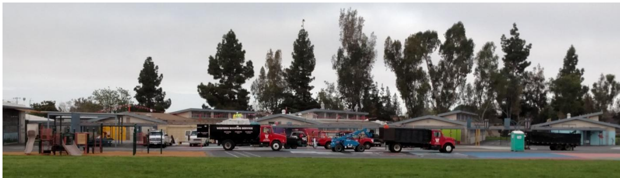
Re-roofing of Russo McEntee Academy- Spring Break 2016
