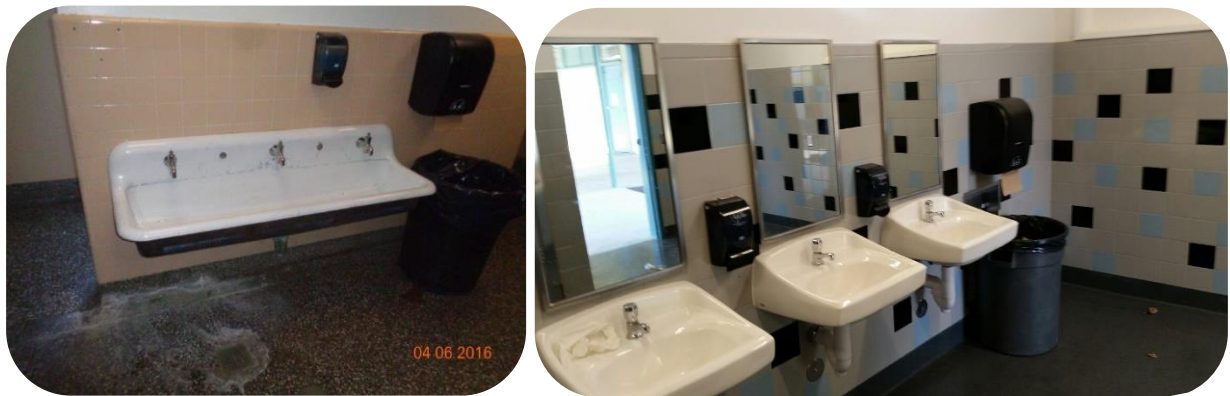
Cassell restroom sinks before and after.
