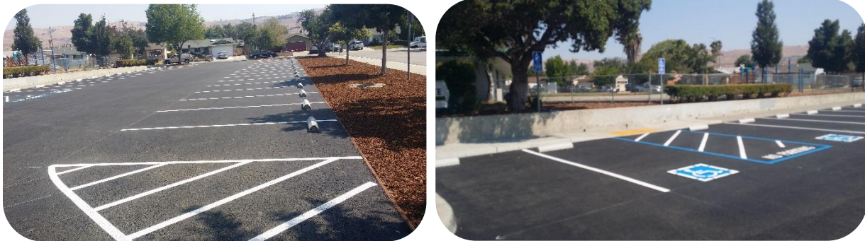
Adelante Paving Project
