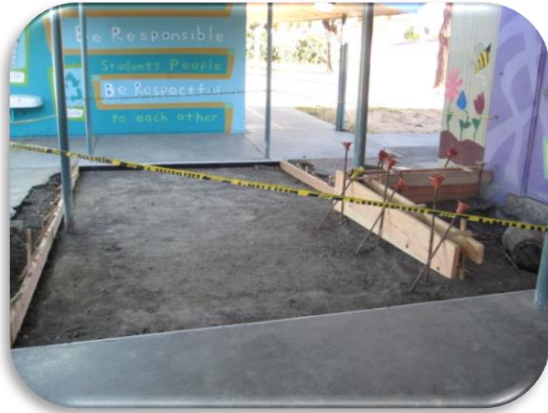
Figure 5 Ryan STEAM Academy (1967) Walkway Construction
