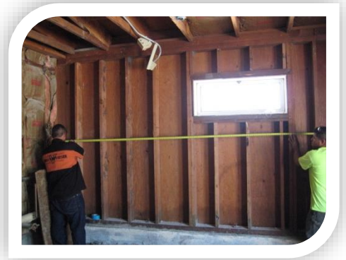
Figure 2 Adelante Dual Language Academy Restroom Renovation
