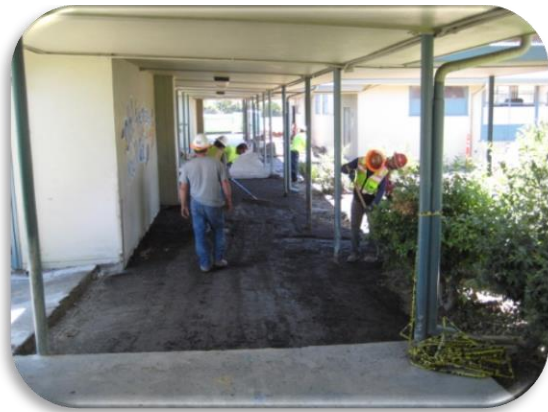
Figure 6 Ryan STEAM Academy (1967) Walkway Construction
