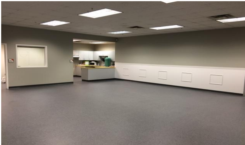
Senior Center Flooring and painting
