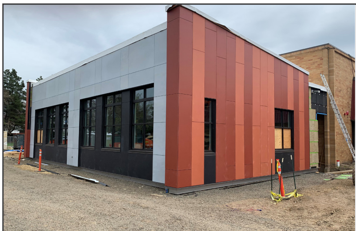
Northeast addition exterior siding
