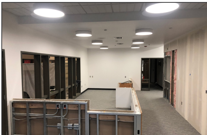
Office reception area
