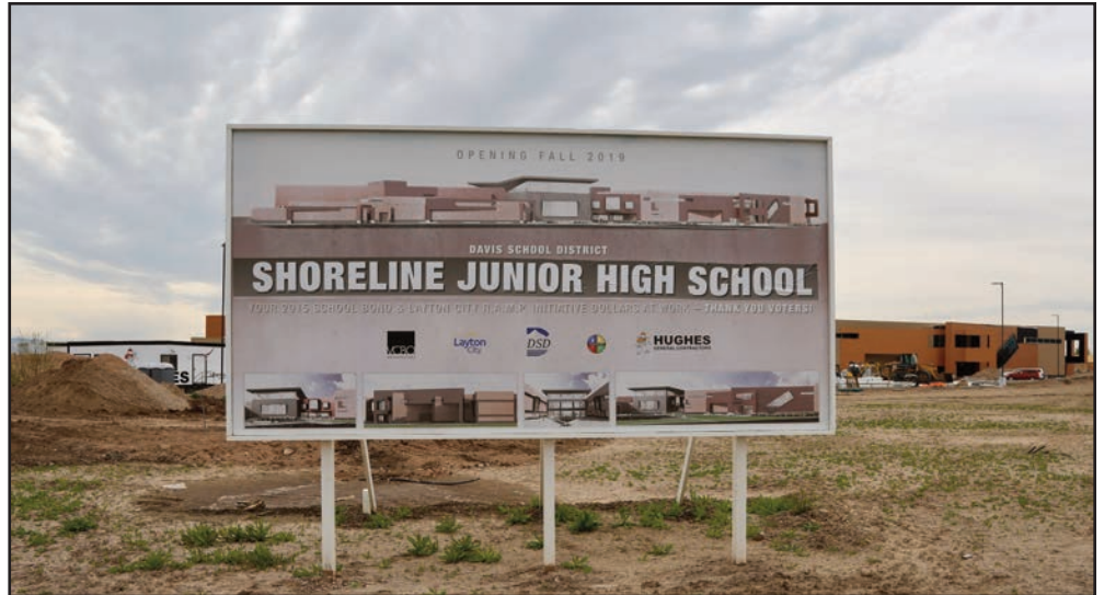
Construction continues at Shoreline Junior High. The project is being funded by the 2015 voter-approved bond.
