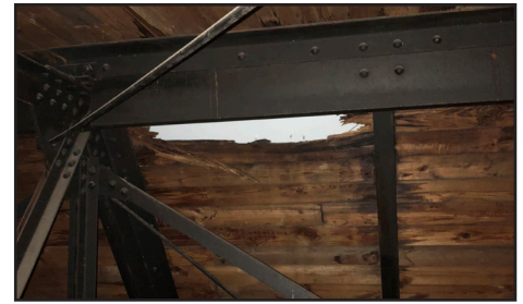
Hole in the roof above auditorium
