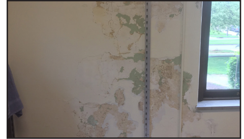
Water damage from roof leak
