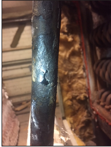
Broken hot water tube
