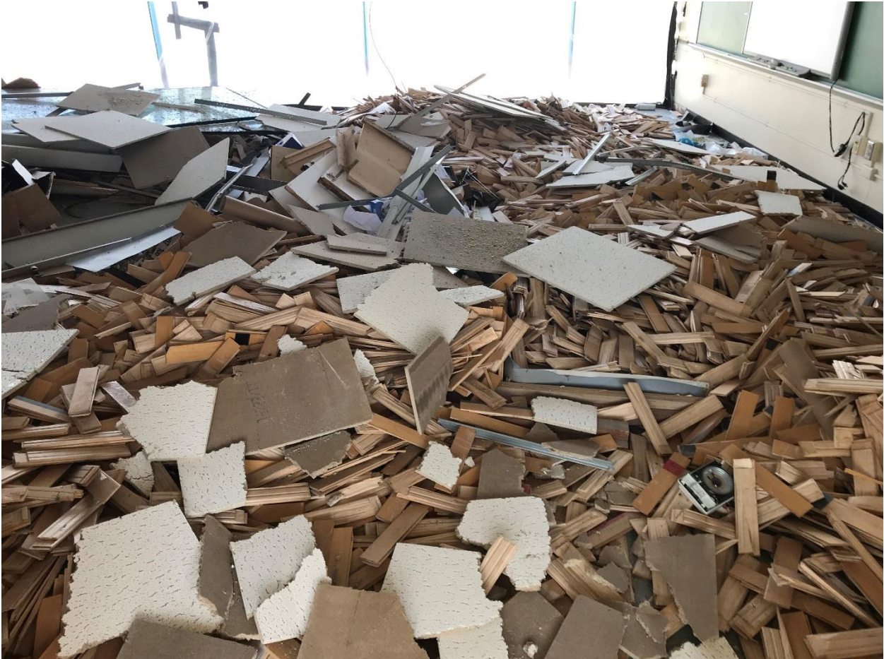
Gymnasium flooring removal – 4/24/19
