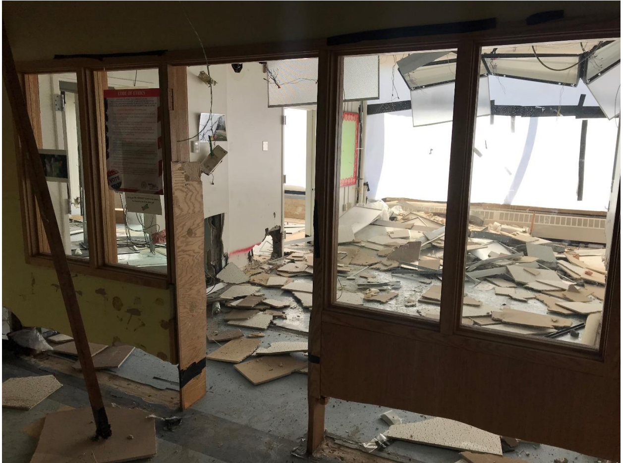
Main Office Abatement – 4/24/19
