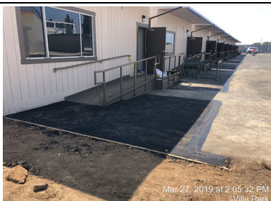
Asphalt landing off of the modular classroom unit ramps.
