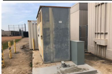
400 Amp breaker added to existing switchgear to power modular units.
