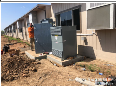
Set new transformer and electrical panel behind interim modular classroom units.
