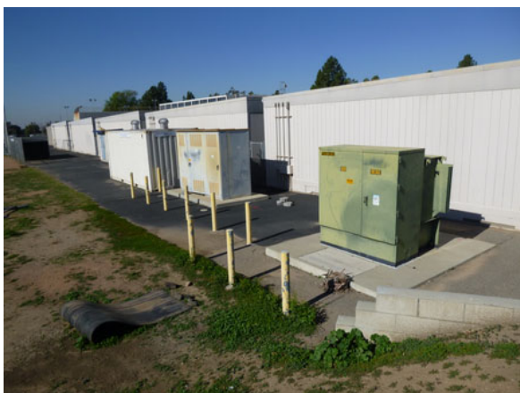
Existing power where the new switchgear will be tie-in to supply power for the (10) Interim Housing modular units.
