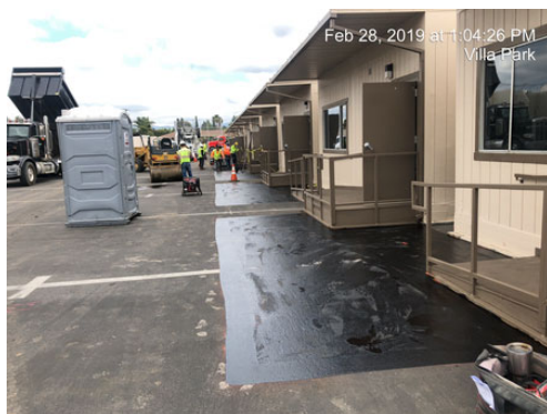
Interim Housing modular set in place and ground prep for asphalt.
