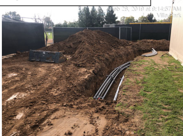
Trenching for electrical conduit behind modular units, near the softball field.
