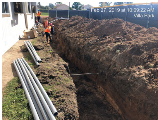
Trenching for electrical conduit behind modular units.
