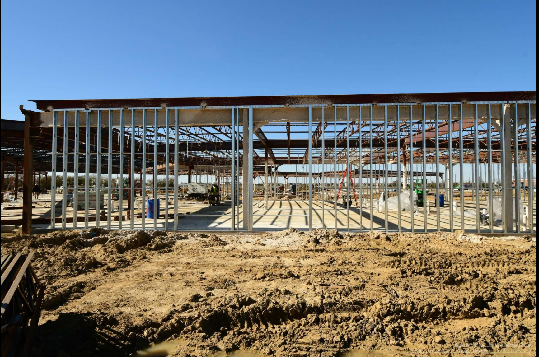
Early Childhood Center Classroom Wing Exterior Wall Framing
