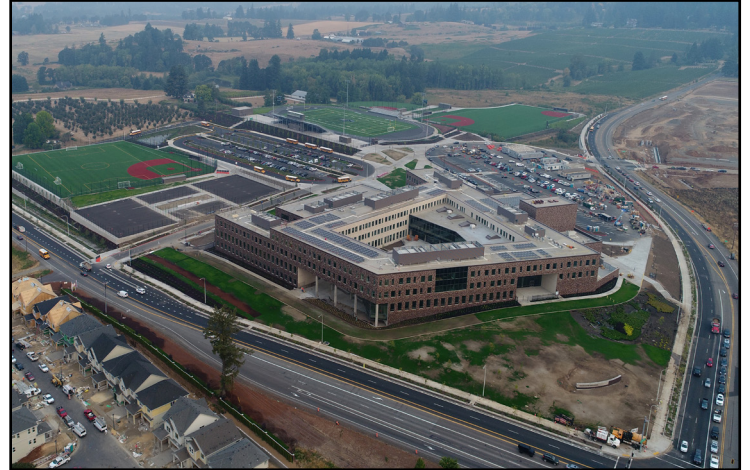
Aerial view looking northwest
