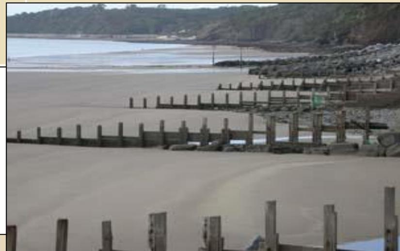
Groynes interfere with the movement of coastal sediments. By trapping sand and shingle, groynes may starve beaches further down the coast of sediment and accelerate erosion there. They are intrusive and look unsightly.
