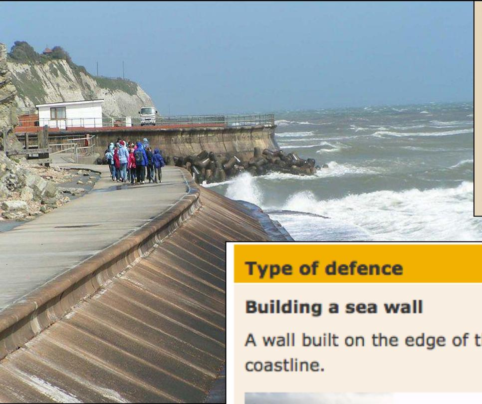
Concrete walls or rock structures built along a stretch of coastline and designed to stop erosion and floods. Sea walls reflect waves, and give complete protection against erosion.
