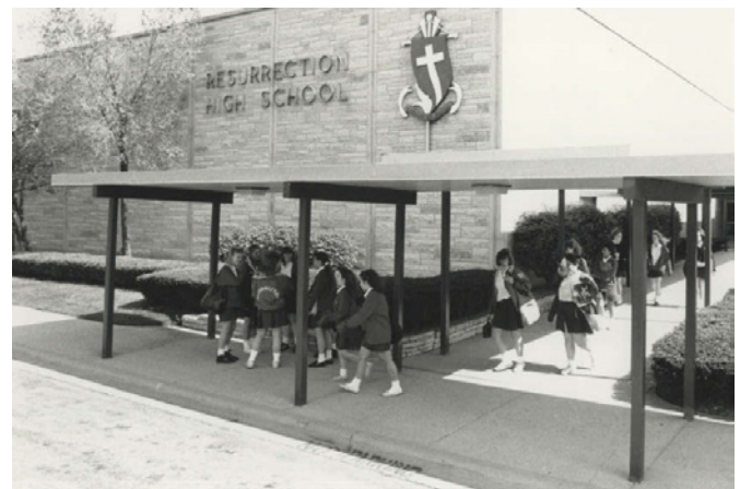
The 1962 school facility opened at Talcott and Oriole.
