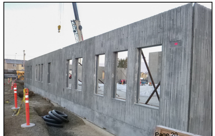
Precast panels in administration area
