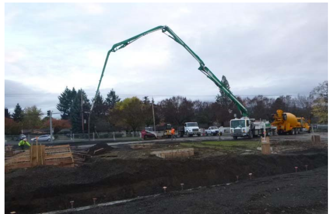
Pouring concrete footings
