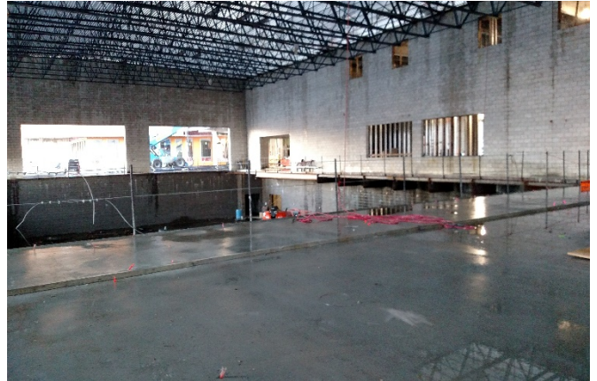
Cement pour of running track around gym
