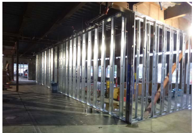
Interior partition framing and rough-in
