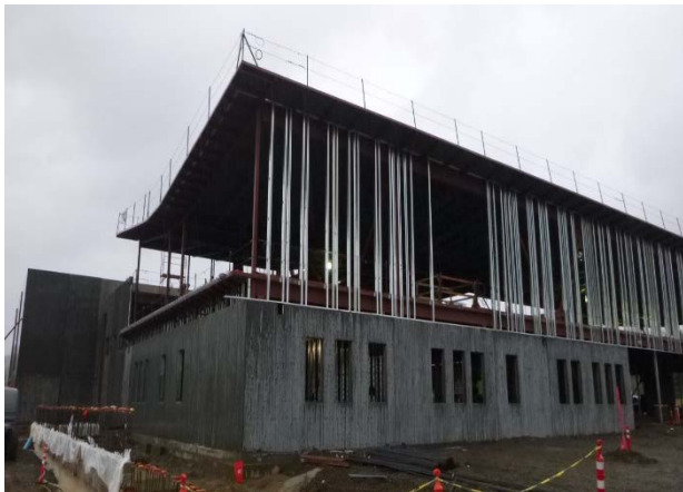
Exterior wall framing
