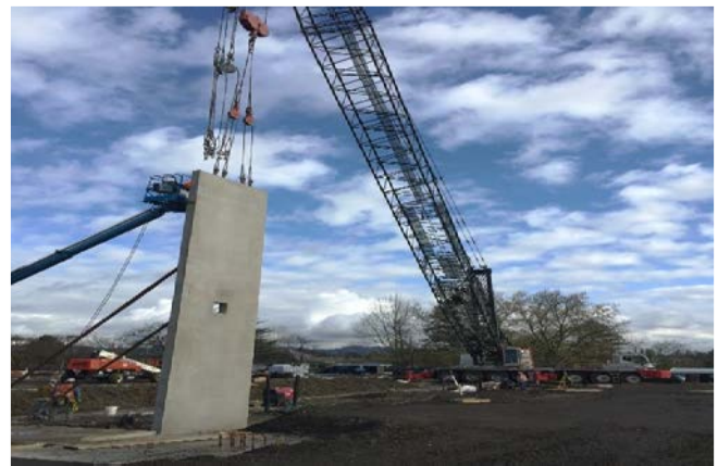
Precast panel installation
