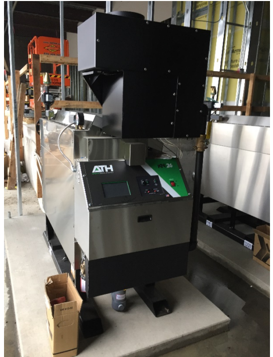
One of Two Condensing Boilers
