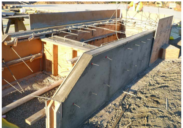
Removal of footing forms
