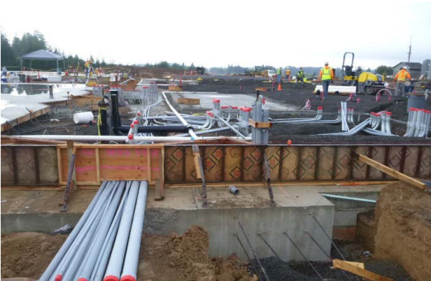
Electrical grid installation
