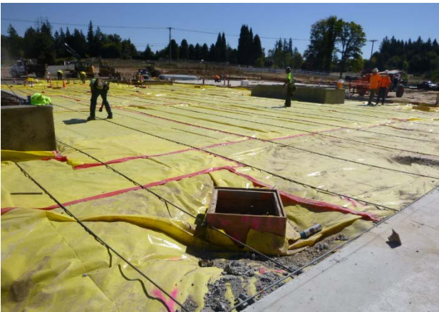
Preparation for rebar
