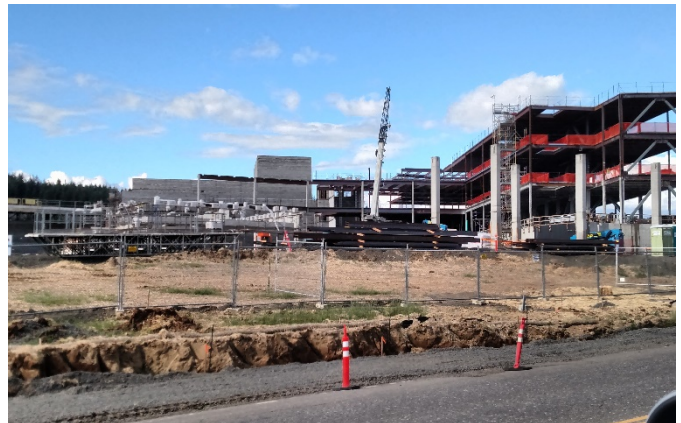
Side View from Scholls Ferry Road - looking north
