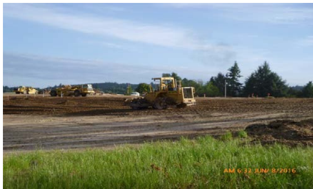
Grading and Excavation - looking northwest
