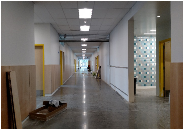
Classroom Wing - looking east
