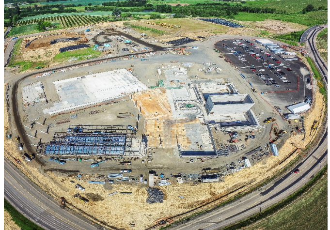
Site View - looking northwest
