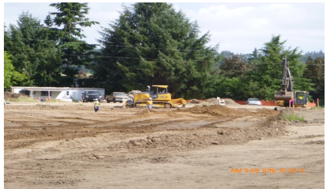
Construction Entrance - looking northwest
