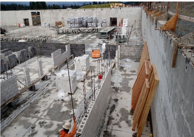
Stairwell/Concessions - looking west
