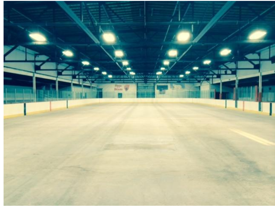
Hippodrome Floor replacement, lighting upgrades, painting
