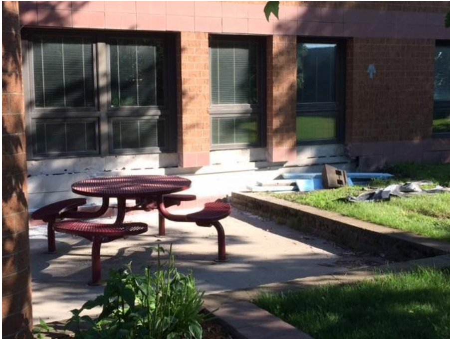
Otter Lake Elementary School Windows and masonry repairs
