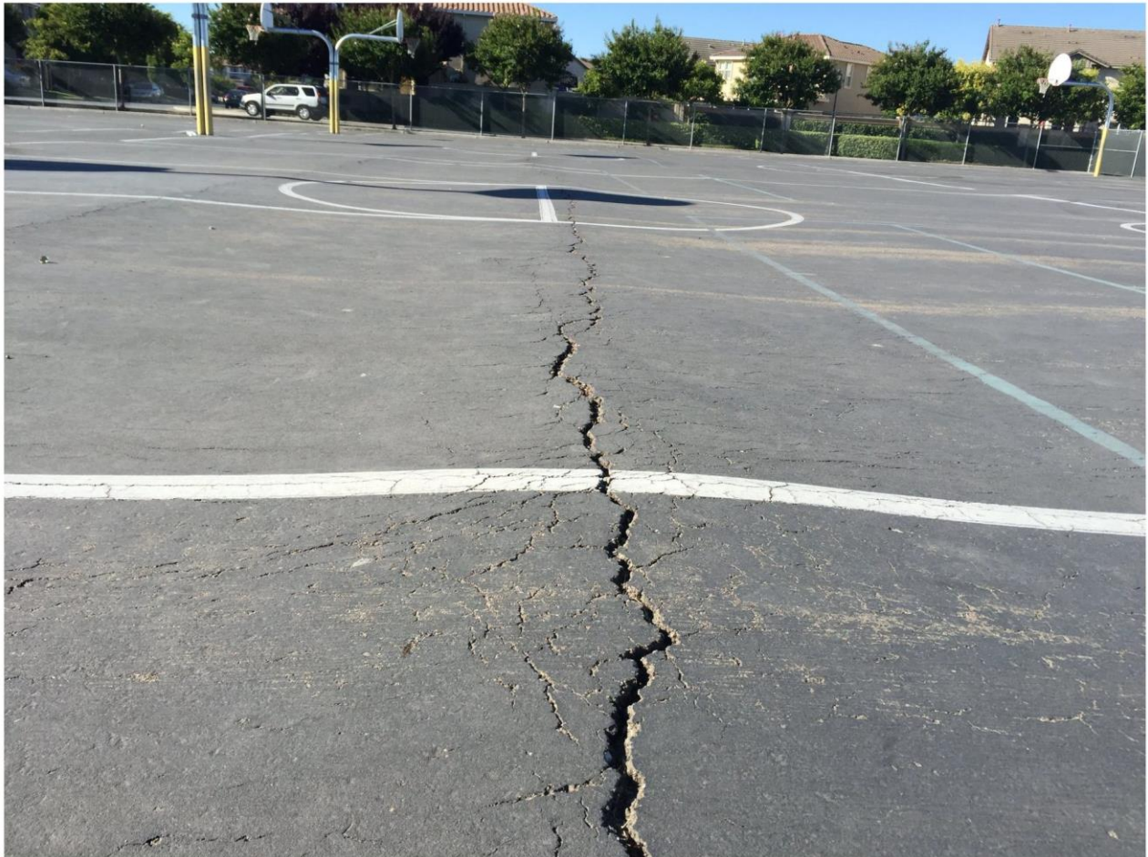
Photo-1: Heaved area running north south across the hardcourt
