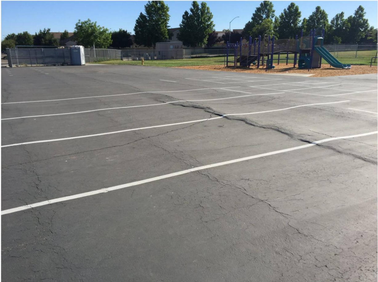
Photo-2: Heaved areas running north south across the hardcourt.
