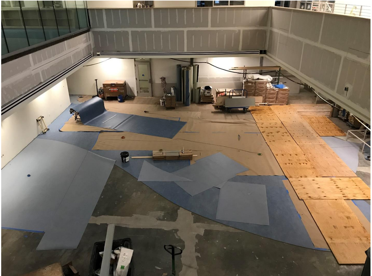
Cafeteria Flooring layout and installation – 1/29/19
