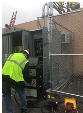
Testing new owner furnished electrical equipment.
