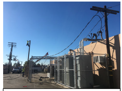
Southern California Edison removing unneeded overhead power lines.
