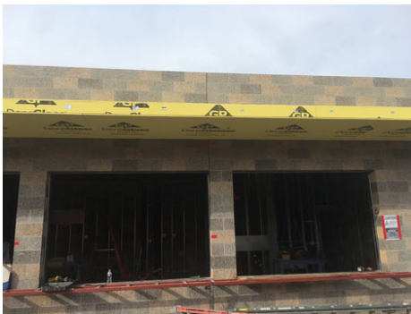
New Satellite Kitchen overhang, serving window and interior wall framing.
