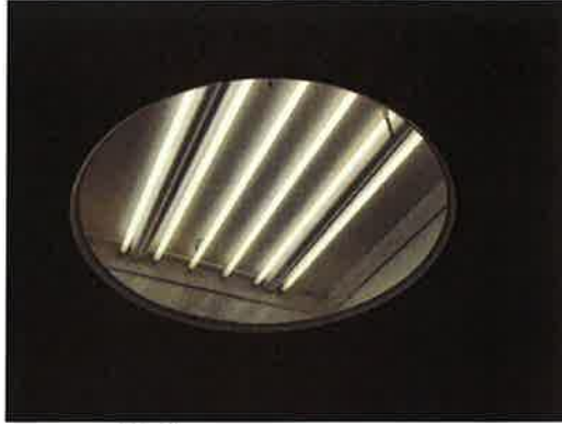
Hallway fixture needs lens
