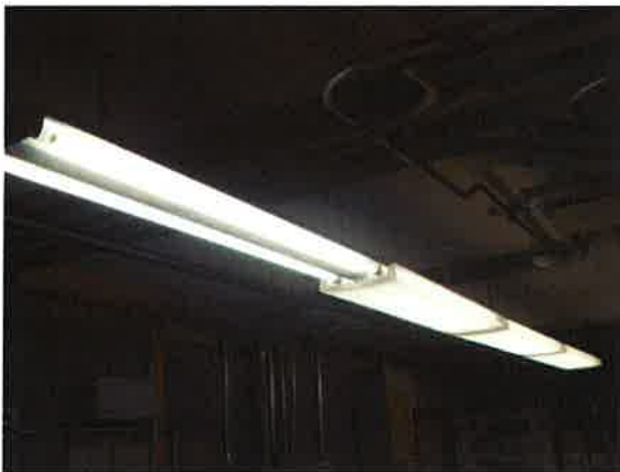
Typical Wraparound Lighting / with Occupancy Sensor
