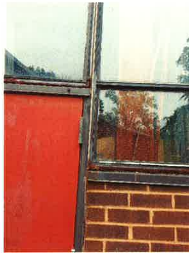
Rusted thru steel window frame
