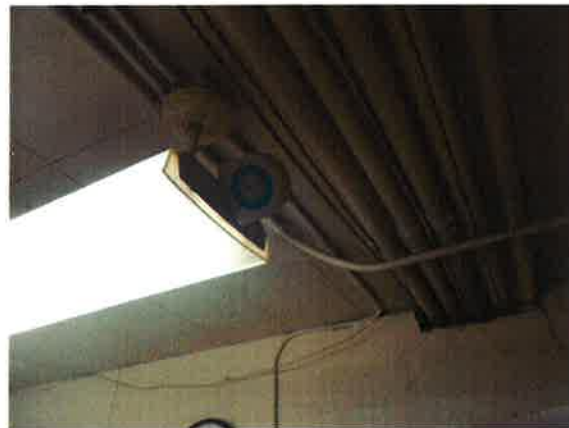
Typical Wraparound Lighting / with Occupancy Sensor
