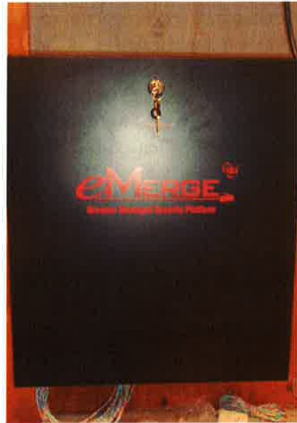
Security Access / Card Reader - Controller
