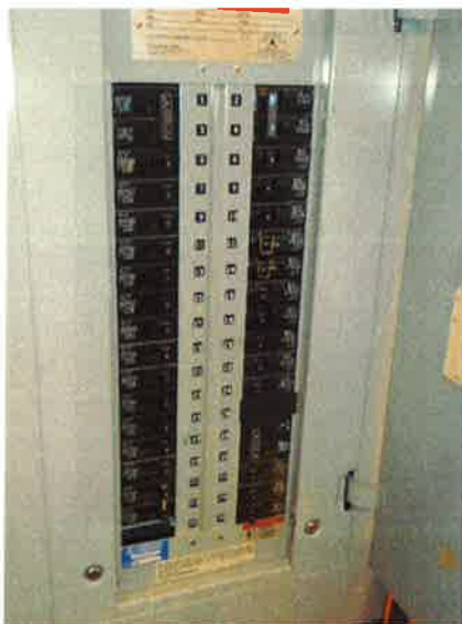
Electrical Pnl (Unlabeled) one circuit available
