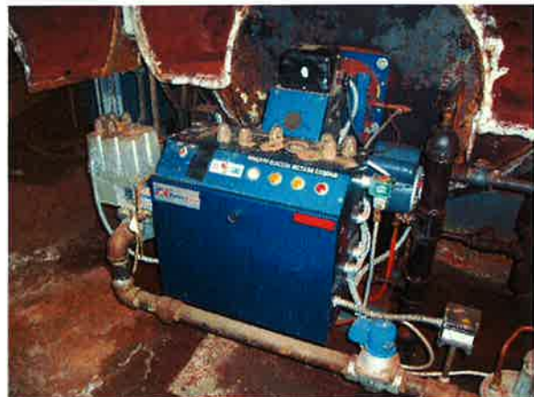
Retrofit burner on original boiler
