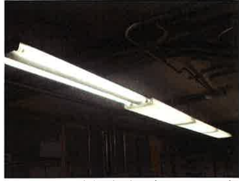
Damaged / missing lens example
