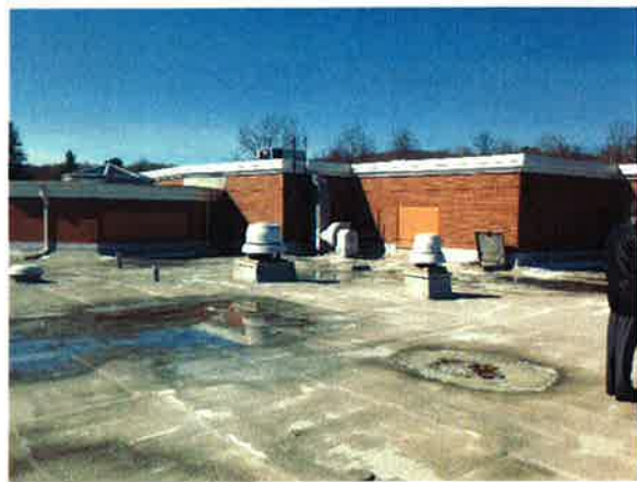
Failed roof toward gym, entry
