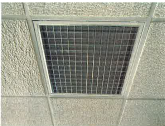
Low glare 2 x 2 fluorescent lighting found in board room
