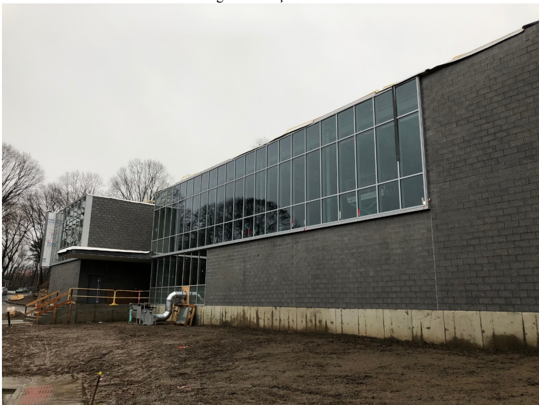
Building North Façade – 12/28/18
