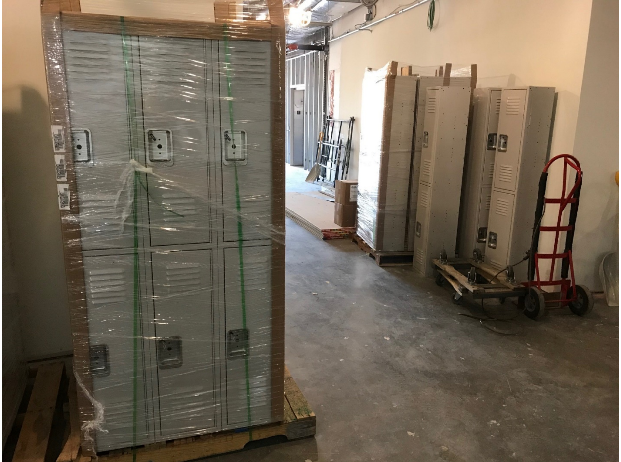
Lockers awaiting installation – 12/19/18
