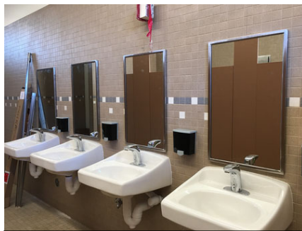
Girls restroom hand sinks, mirror, fixtures and accessories set in place on wall.
