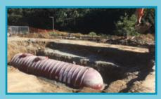
The Mile Creek oil tank installation (pictured) is nearing completion. After the old tank was removed, some blasting was necessary to make sure room was available for the new tank. This is the final project in our three-year-cycle of oil tank replacements and is expected to last 30 years before having to be replaced again.
