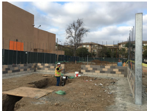
Electric Yard conduit and vault prep and masonry block course for the building.
