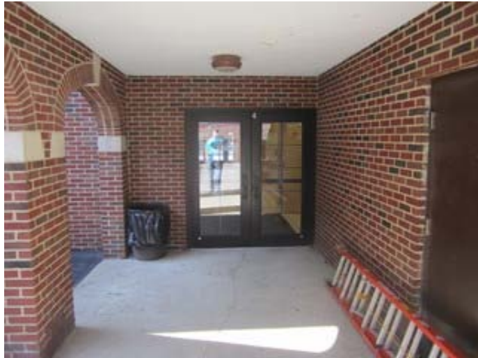
Aluminum Exterior door in 1968 Addition
