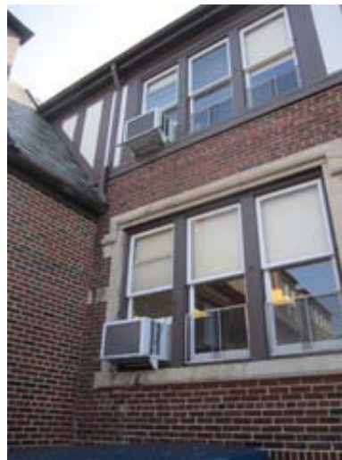
Windows of 1968 Addition
