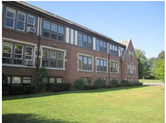
Exterior Wall at Joint of Original Construction and 2003 Addition
