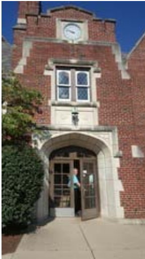
Wood Exterior Door in 1928 Original Construction
