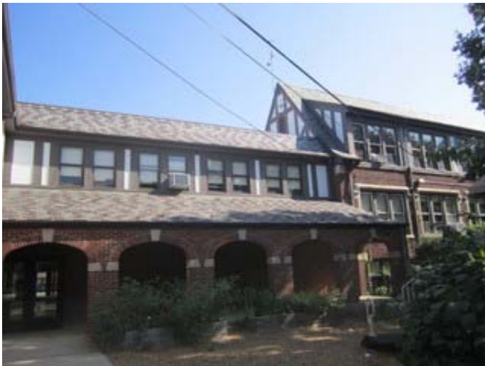
Exterior Wall at Joint of Original Construction and 1968 Addition
