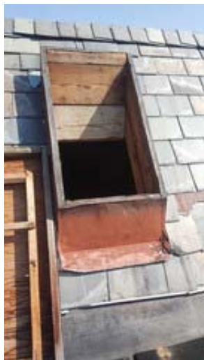
Original Roof Hatch Over the 1928 Original Construction
