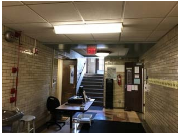
Typical Corridor Lighting
