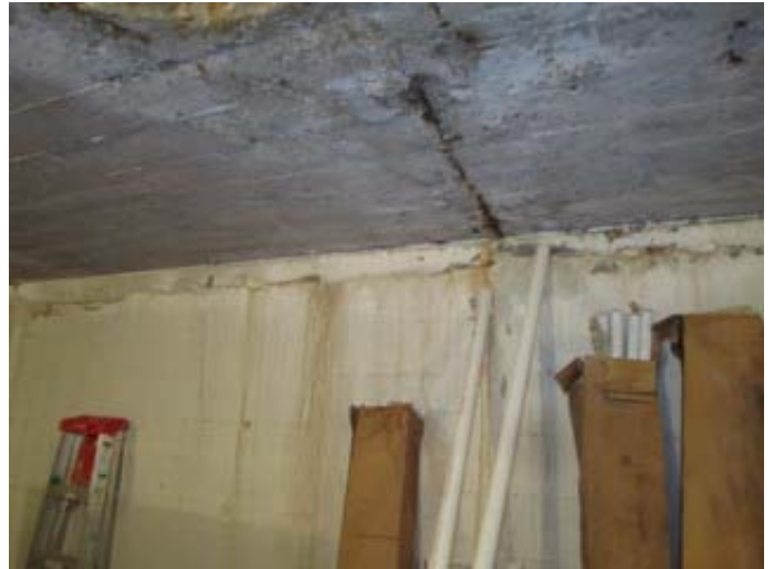
Foundation at Abandoned Coal Chute
