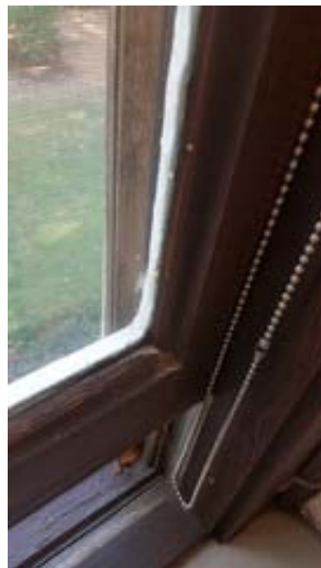
Window of 1928 Original Construction
