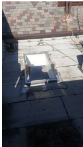
Skylight in 1927 Original Construction
