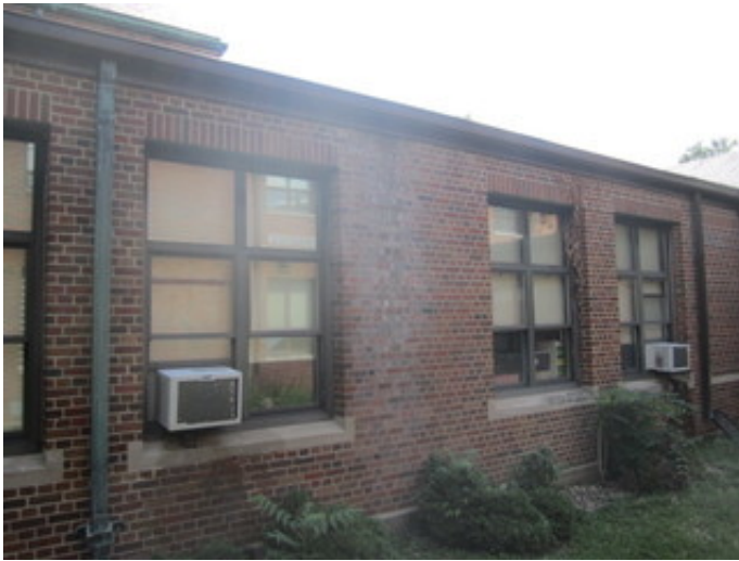
Courtyard Elevation of 1932 Addition
