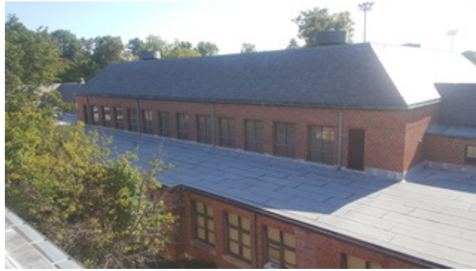
Roof Over the 1932 Addition
