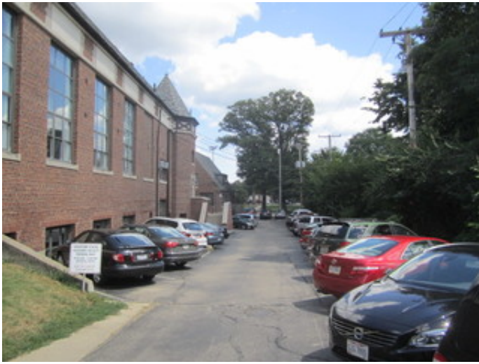
Staff Parking Lot
