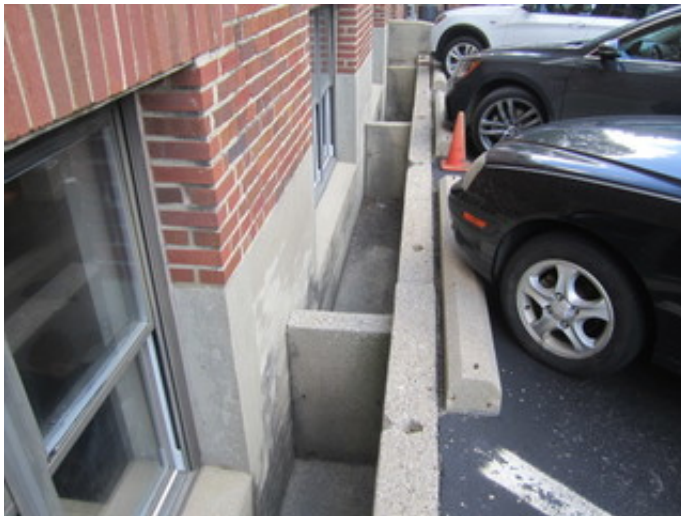
Foundation at 1927 Auditorium Construction
