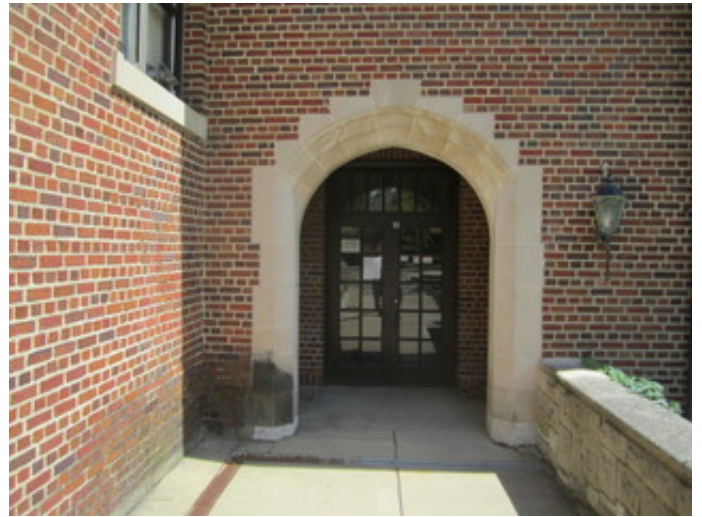
North Entry of 1927 Original Construction
