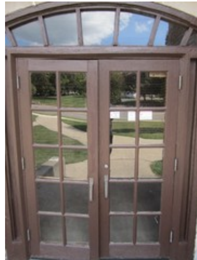
Typical Entrance Door
