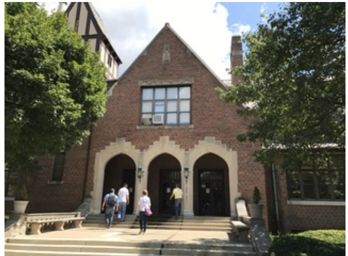
Exterior Lighting At Entry
