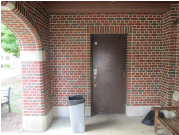
Typical Exterior Door
