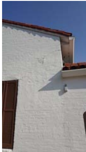
Masonry Wall on South Elevation
