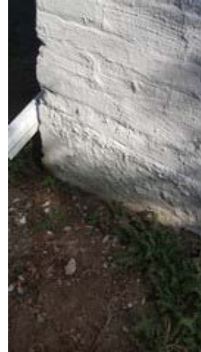
Exposed Foundation Wall
