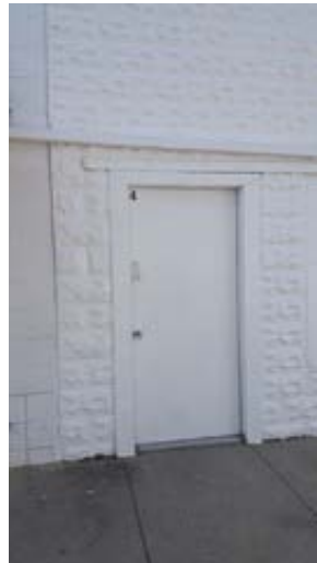
Control Joint at Dissimilar Materials
