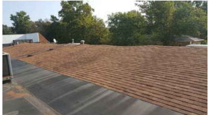
Membrane and Asphalt Shingle Portion of Roof
