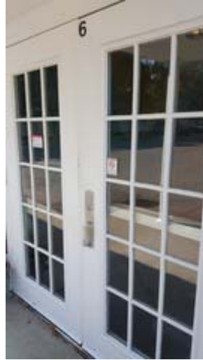
Typical Entrance Door
