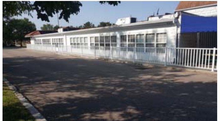
Windows in East Elevation
