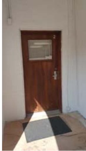
Typical Exterior Door
