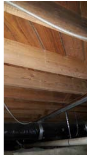
Floor Framing above Crawl Space
