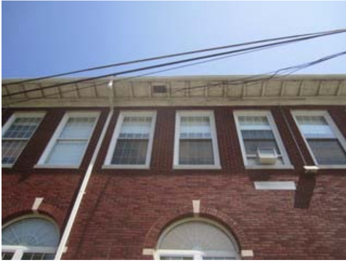
Soffit at 1949 South Elevation
