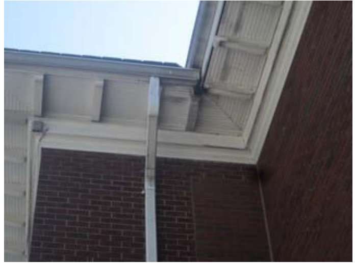
Soffit at 1949 and 1909 Intersection
