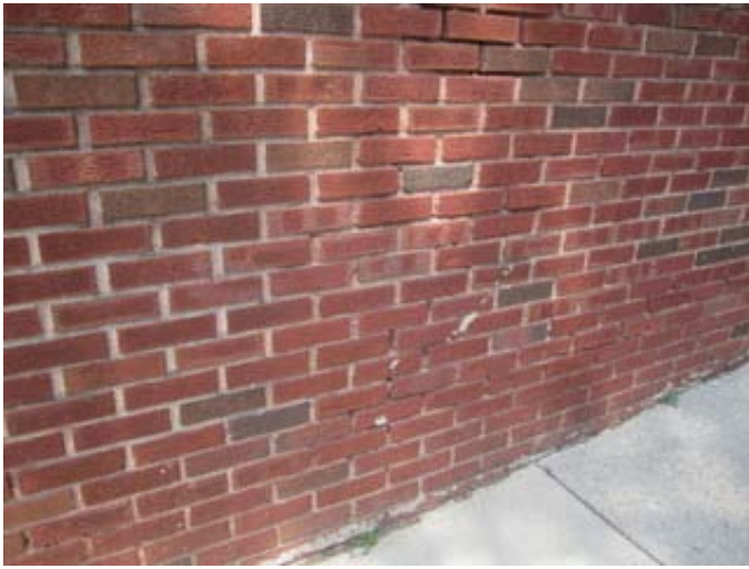
Base of Exterior Wall of 1949 Addition
