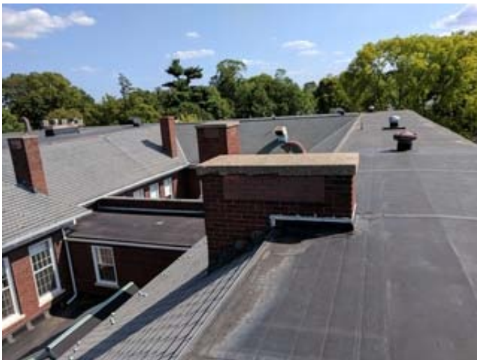
Existing Roof Over 1909 Original Construction
