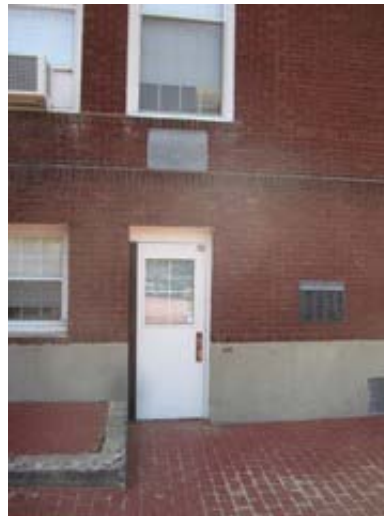
Typical Exterior Door
