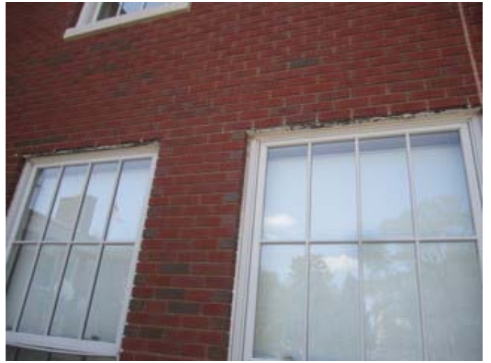
Steel Lintels at 1949 Addition
