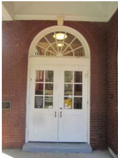
Typical Entrance Door
