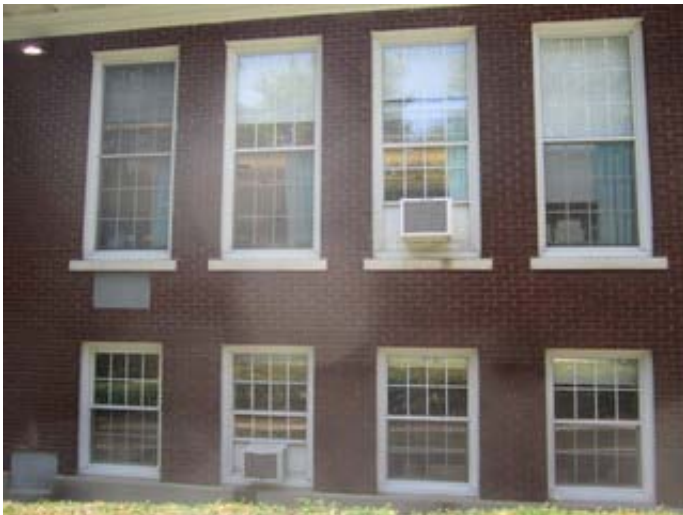
Windows at Entry Courtyard
