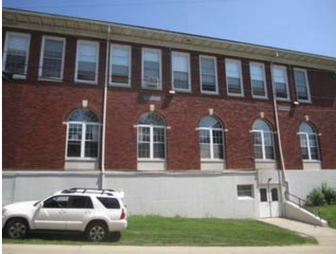
West Elevation Foundation Wall
