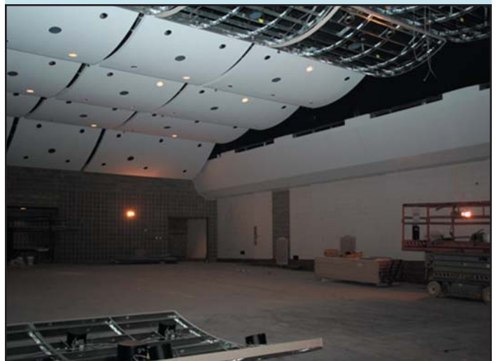
Victor Junior/Senior High School Auditorium Ceiling Cloud Construction, May 2007
