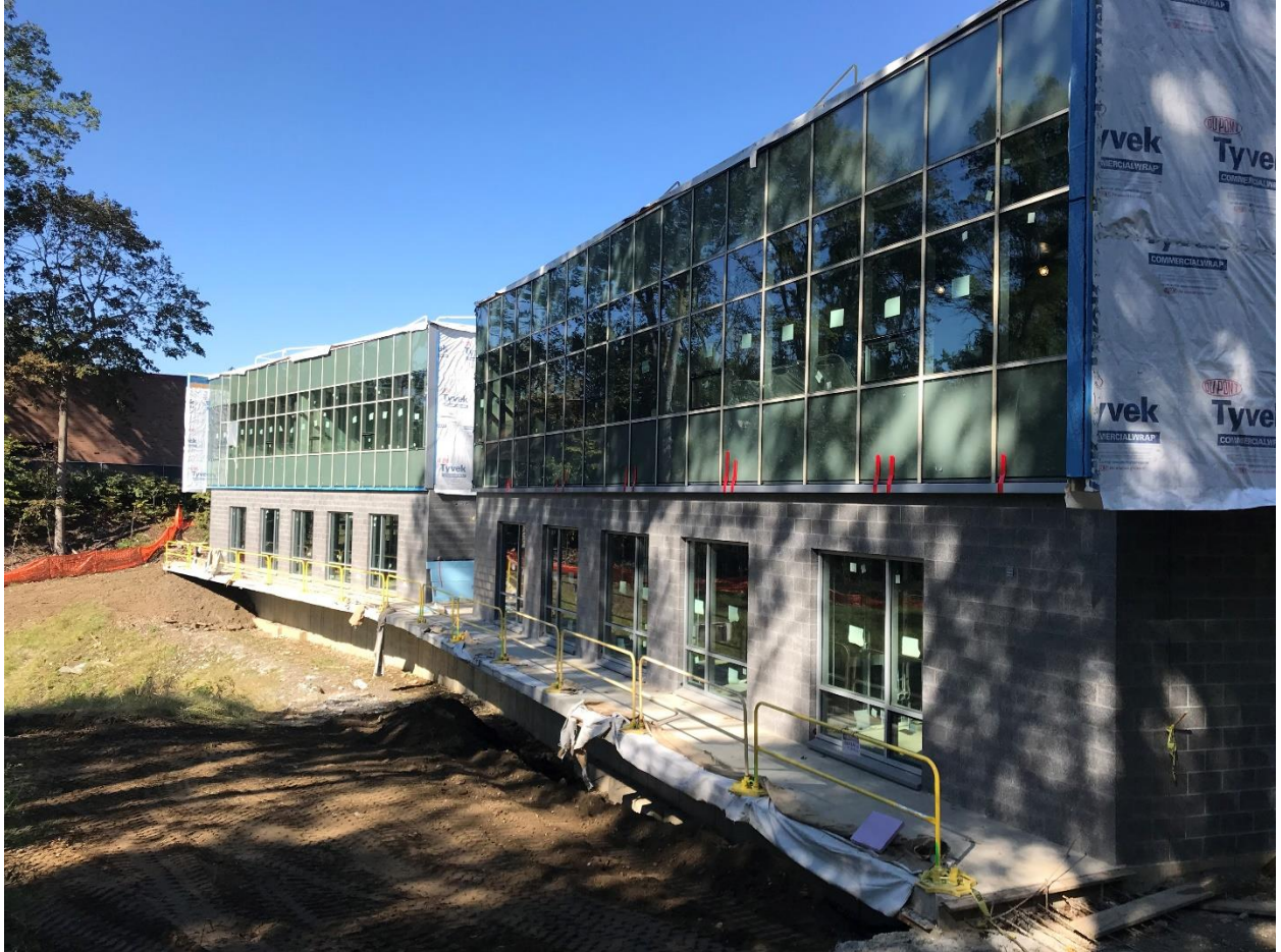
Building South Façade – 10/17/18
