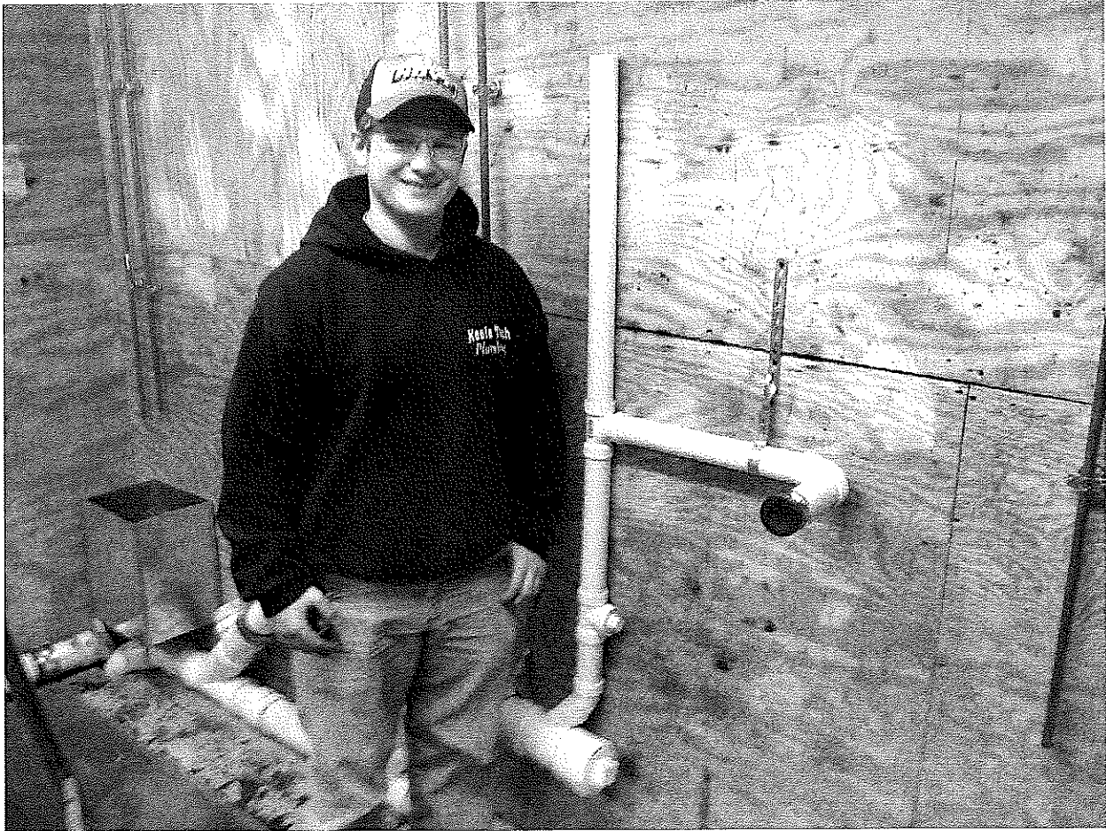
Keefe Tech Plumbing Senior Michael Sweeney of Framingham standing next to the house drain assembly he installed.
