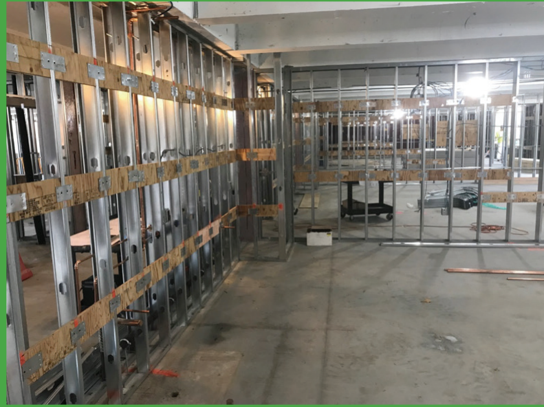
2 ND FLOOR FRAMING AND IN-WALL ROUGH-IN
