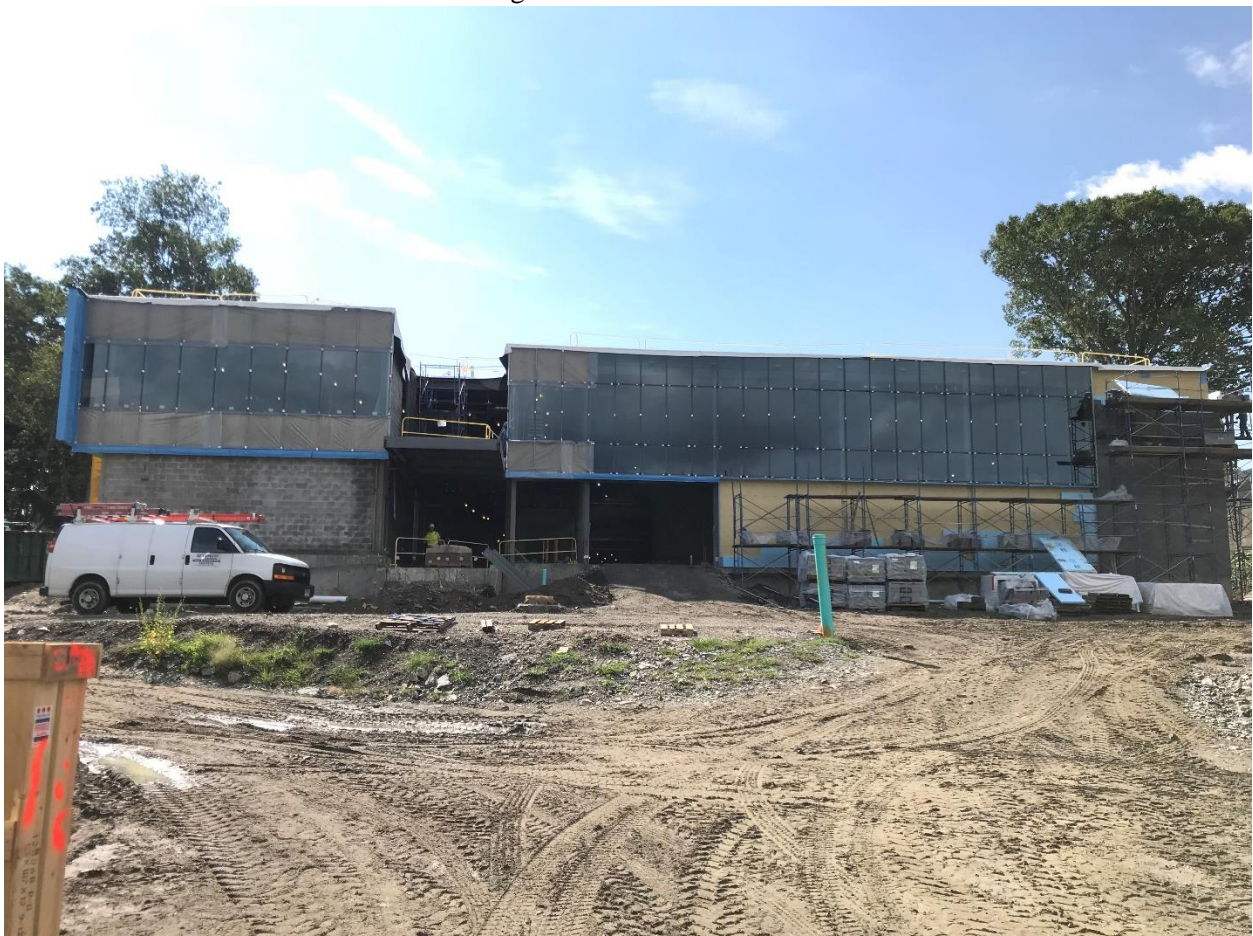
Building North facade – 9/19/2018
