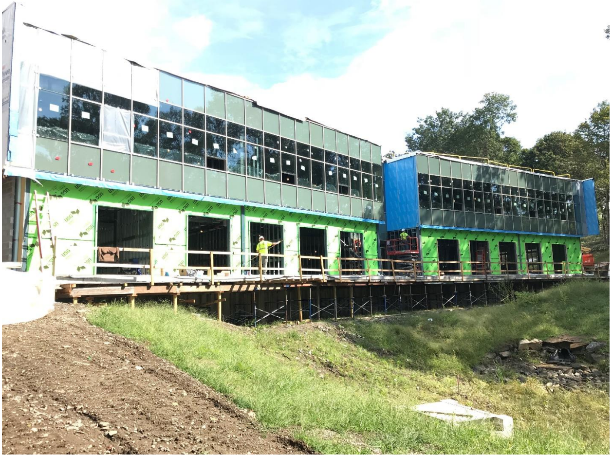
Building South Façade – 9/19/18
