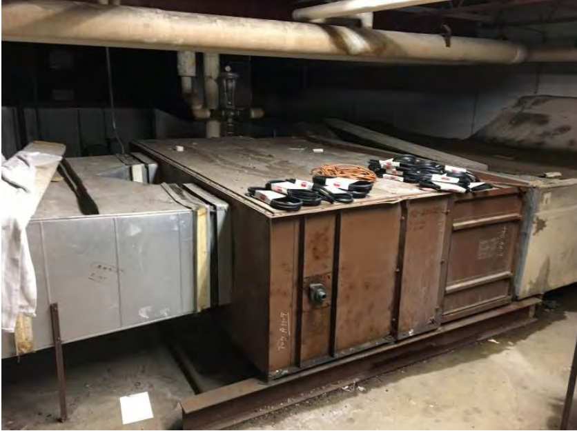
electrical centrifugal chiller manufactured in 2003 by McQuay. This chiller has a capacity of 1,100 tons.
