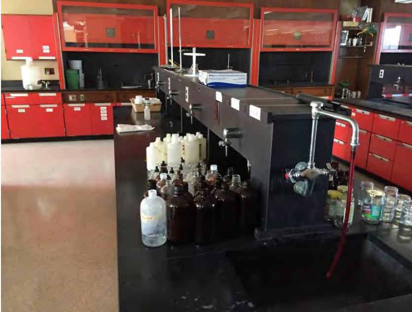
the gang type with master mixing valve assembly.
