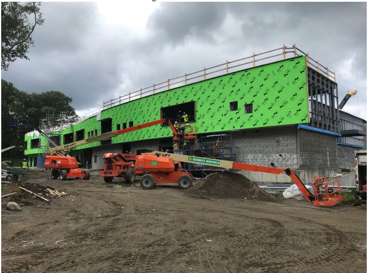
Building East facade – 8/18/2018
