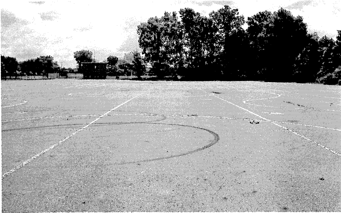
Photograph No. 1 From Boring B-12, facing south.
