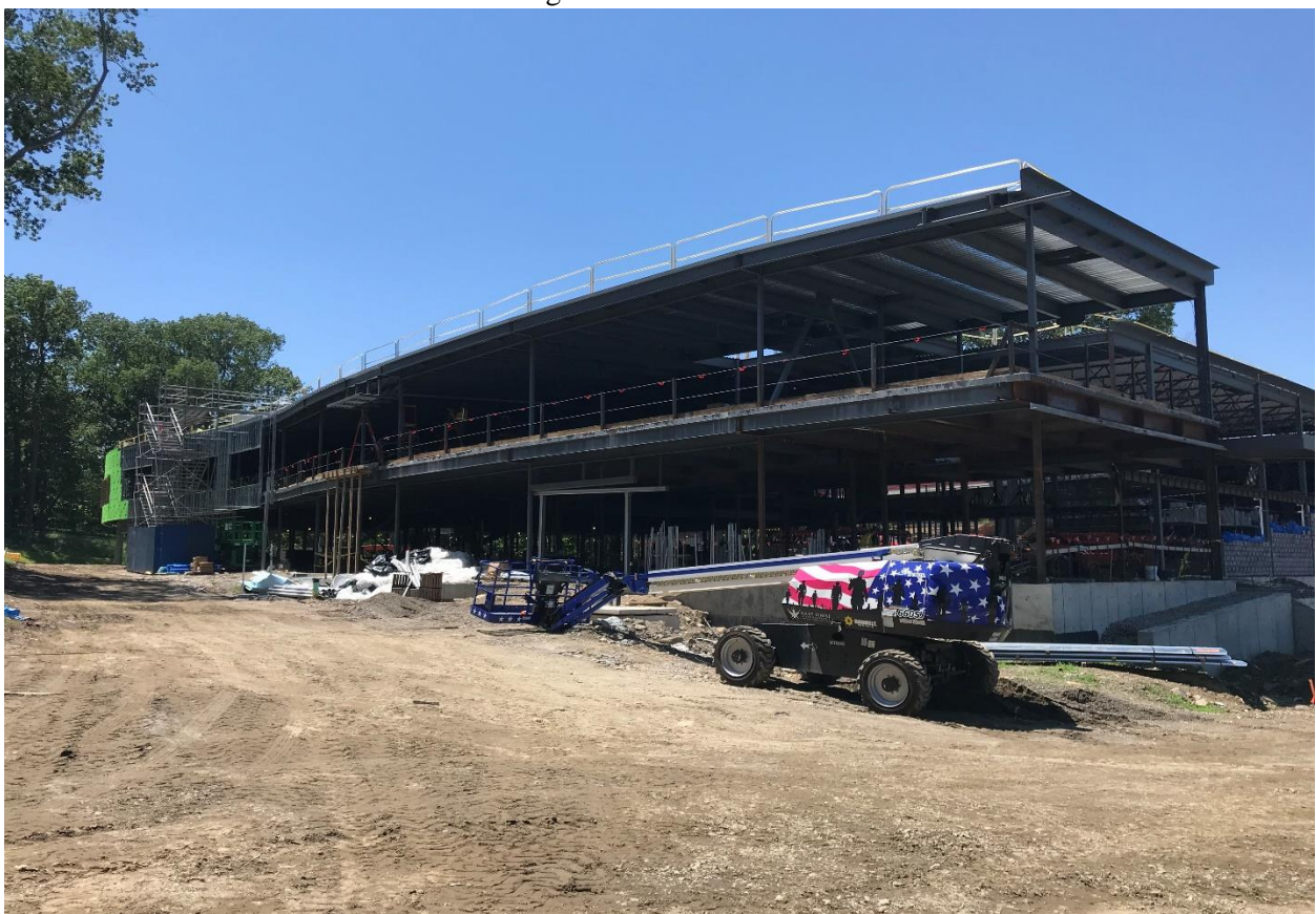
Building East facade – 7/18/2018
