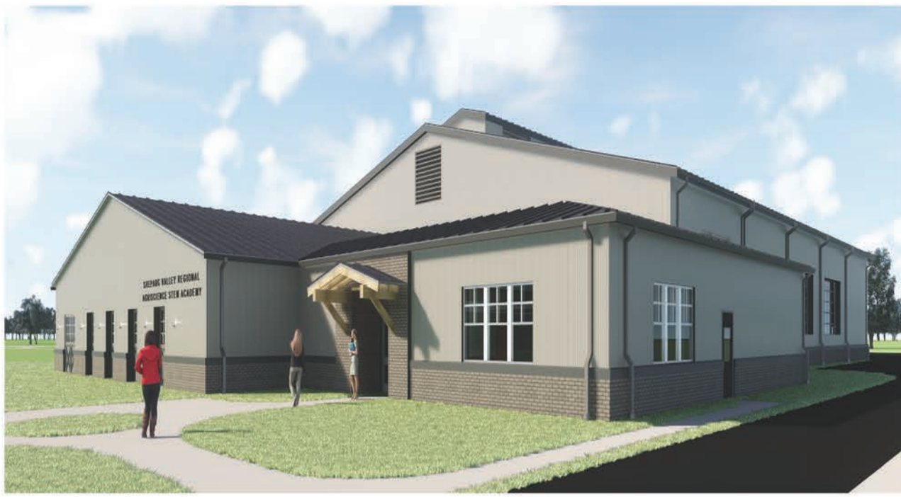
EQUINE / GARAGE / ANIMAL FACILITY
