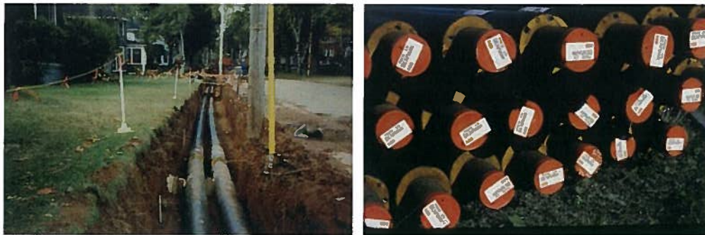
Figure 3 Underground Insulated district energy piping 1
