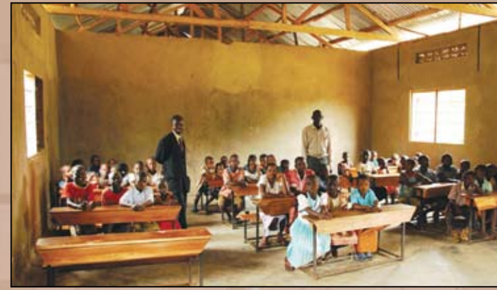
For the Children's Sake Foundation provided funding to build this classroom at Amazing Grace, a school in rural Uganda. The walls and floors are finished in concrete to help keep the dust down.
