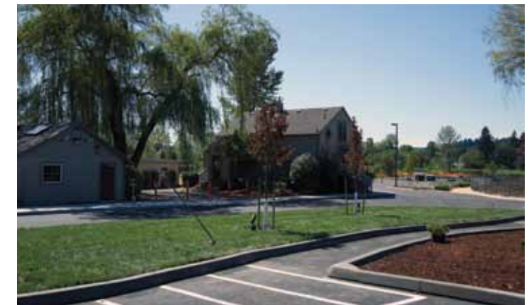
The new Valley Campus parking lots are paved and landscaped. Students enjoy recess on the expanded playground while new fencing improves security.
